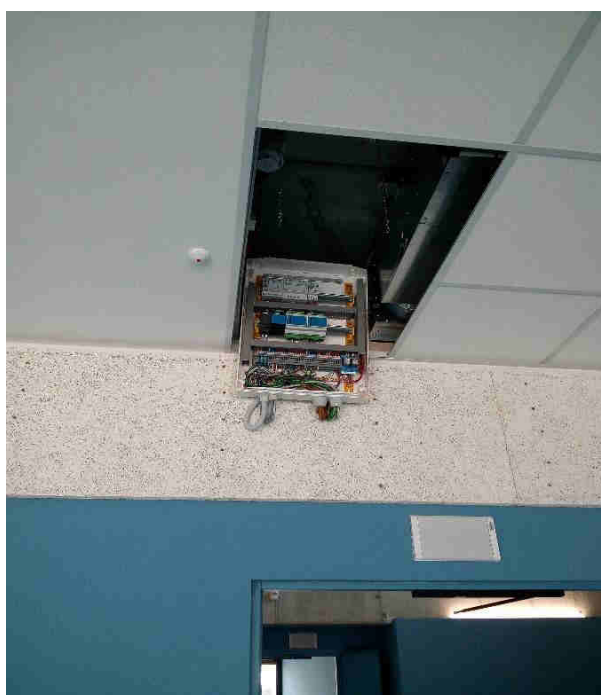
Fig. 11. The AHU adjustment panel of the class.
